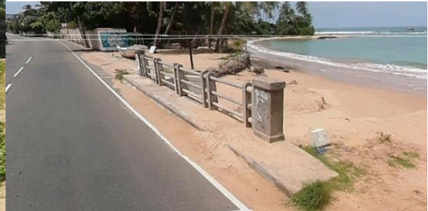
Exhibit 4: Outlets of Tuduwegoda canal (a) Mawakada canal (b) are filled with sand
