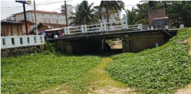
Exhibit 4: Outlets of Tuduwegoda canal (a) Mawakada canal (b) are filled with sand
