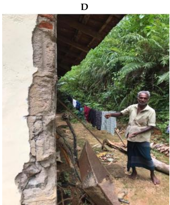
Figure 06: Houses for the landslide risk in the study area
